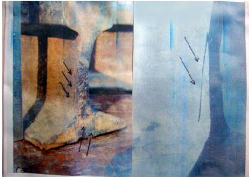
Fig;2.1 Tool mark - Sliding tool marks on railway track
